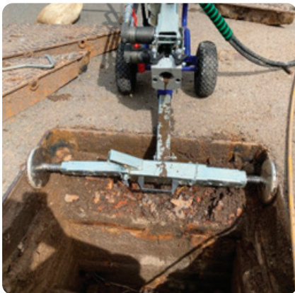
Clamping unit used Horizontally with clamping feet screwed out to secure the machine to the manhole/chamber.
