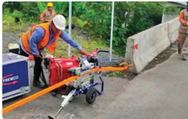
DuctRod RAPID in use pushing the micro duct into the concrete barrier a distance of 280m/306yds.
