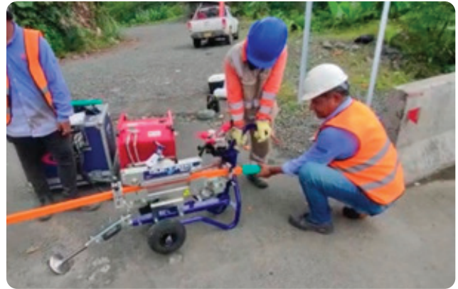
DuctRod RAPID set up with micro duct between chains being guided into the barrier by a technician.
