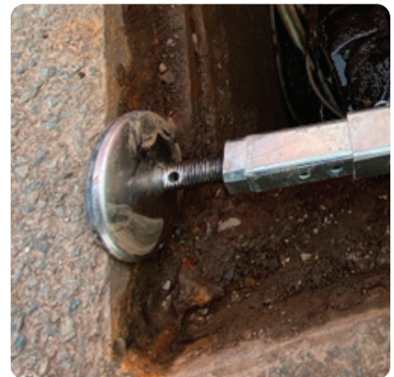
Showing foot screwed out with hole drilled and flat surface for using an adjustable wrench or a screwdriver to turn the shaft that pushes the foot onto the chamber/manhole wall.
