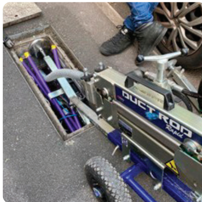
Clamping unit used vertically with clamping feet securely screwed out securing the machine into the smaller chamber/manhole.
